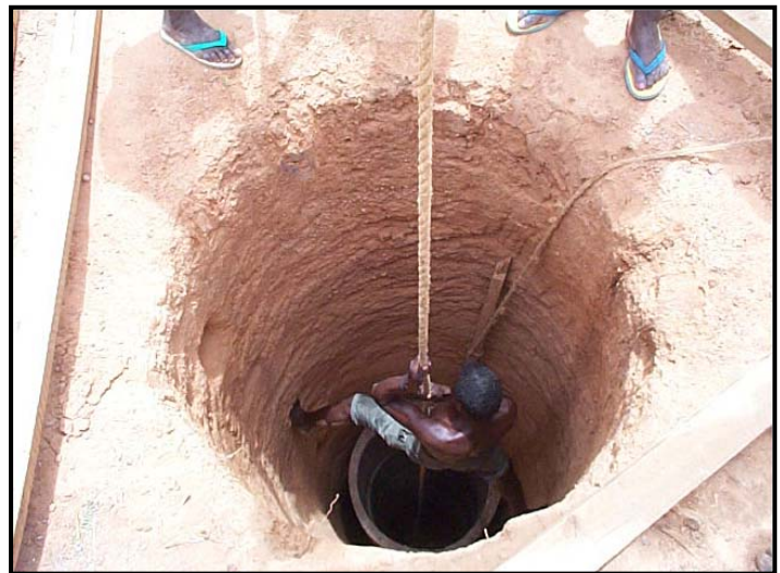
Digging of shallow wells in Garissa
