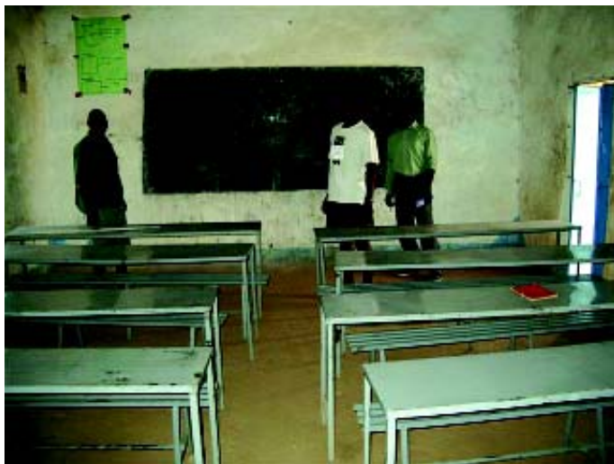
Renovated classroom in Tima School
