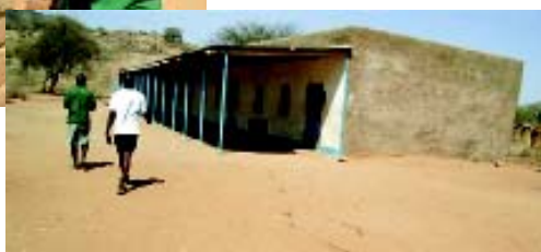
Renovation of Tima School in Nuba Mountains
