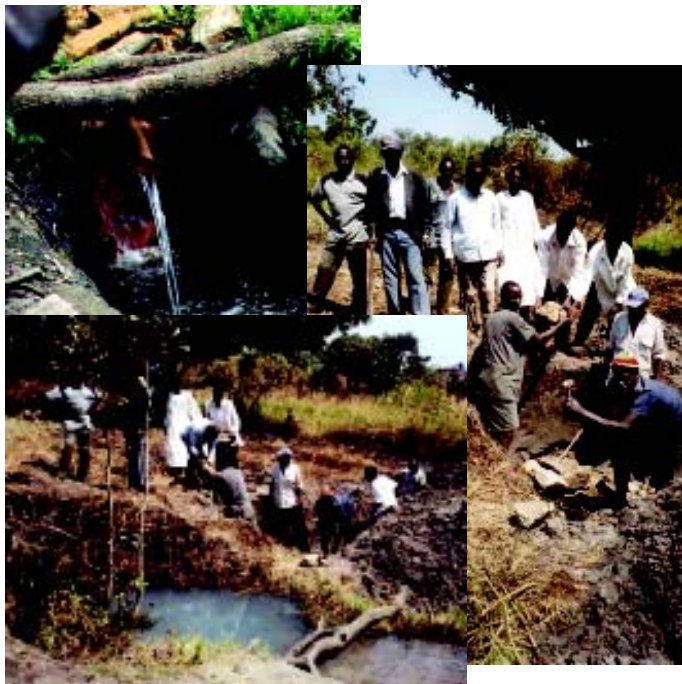
Construction of protected springs
