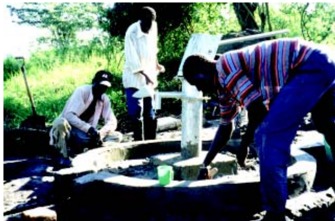
Construction of a pump platform
