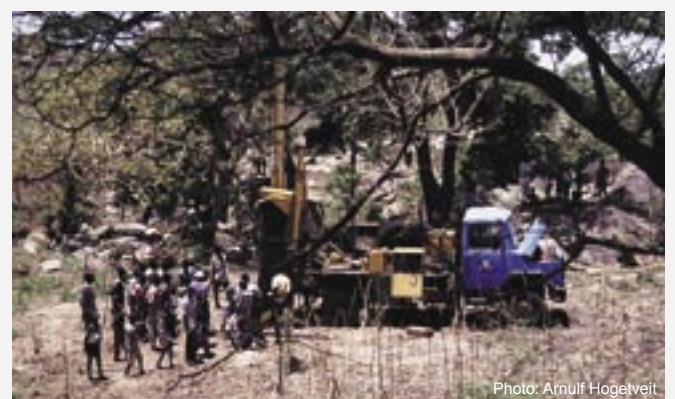
Drilling of boreholes in Northern Uganda . . .
